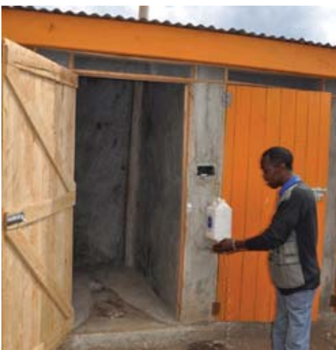
Njogu shows the hand washing feature built alongside a new latrine.
