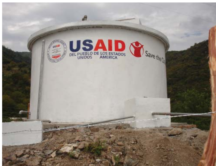
A community helps rehabilitate its water system.
