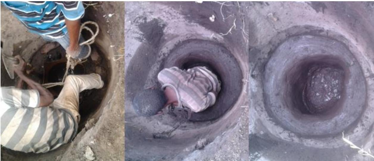
Figure 4: soil cement mixture pit lining
