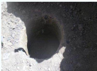
**1.** The pit hole is not deep (0.5m). The contents are made into a small wall around the hole.
