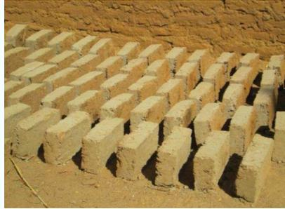
2. Bricks are made to stabilize the pit hole. Good quality sand, cement and brick treatments must be ensured.
