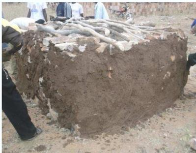
4. The stones are stabilized with the mixture of mud, cow dung and engine oil.
