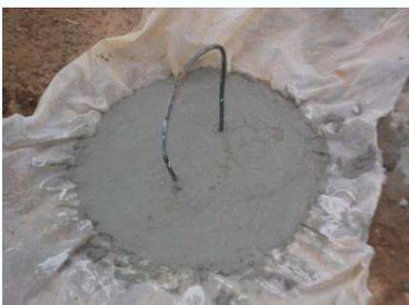
8. A cover for the defecation hole is made.
