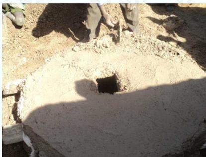
**5.** The slab is consolidated with a mixture of mud and cow dung.
