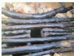
*Wood covered with engine oil to protect from termites and leaking*
