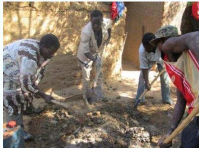
5. Then slab is consolidated with a mixture mud, cow dung and engine oil.
