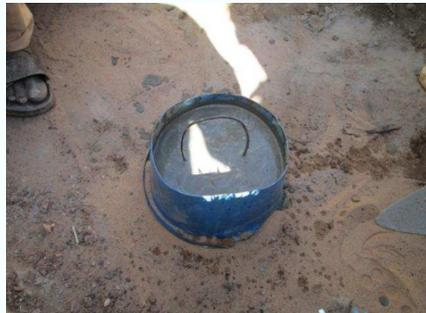
8. The cover is made from a mixture of cement and sand in a hand crafted mold.
