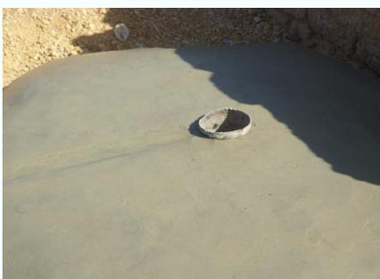
7. If the household has the means a layer of cement can be added to further stabilize the latrine and prevent water infiltration.
