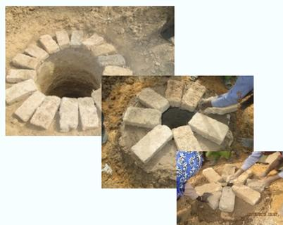
**7.** For the model without wood, bricks are stacked upward giving a conical shape at the top.
