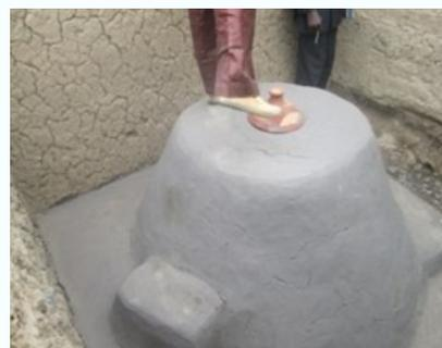
**9.** The surface is made very smooth with mud or cement, one step is added and a cover fabricated.
