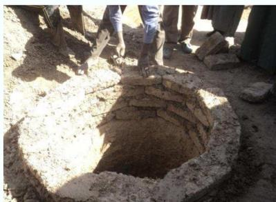
**2.** An extension is built around the pit hole with bricks.
