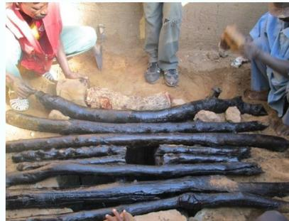
4. The wood of the slab is coated with engine oil to protect it from termites and leaking water.
