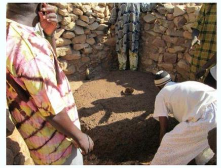
6. Then everything is covered with the mixture prepared at step 2 to prevent water leaking from the slab top.
