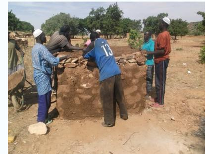
**6.** Then everything is covered with the mixture prepared at step 2 to prevent water leaking from the slab top.
