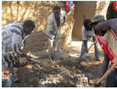
5. Then slab is consolidated with a mixture mud, cow dung and engine oil.
