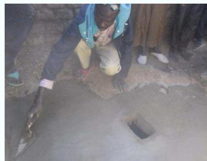
**6.** A layer of cement is added to prevent water from leaking through.
