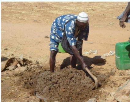
4. A mixture of mud and cow dung is prepared to cover the pit hole.
