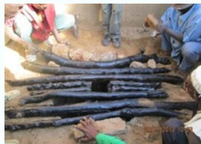
**3.** A wooden slab is prepared and coated with engine oil to protect the wood from termites.
