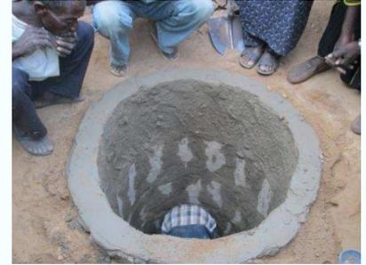
3. The inner walls of the pit - from top to bottom - are stabilized with bricks.
