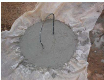
7. The cover is built with a mixture of cement and sand.
